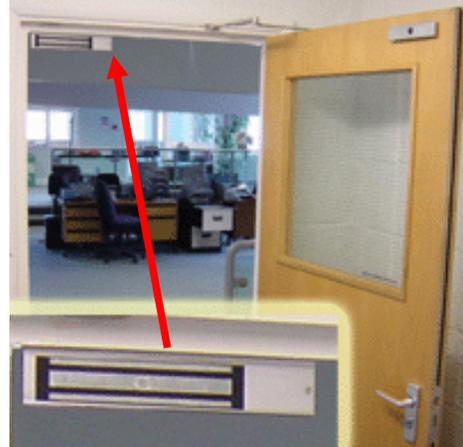
The magnetic lock is mounted on door frame
